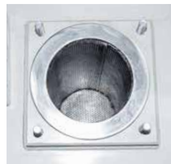
Installed inox filter.
