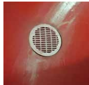
Waste water drain filter.
