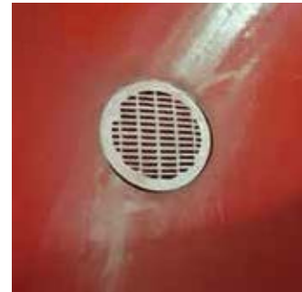
Waste water drain filter.
